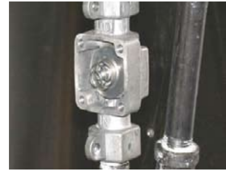
8. New spring/magnet assembly installed.
