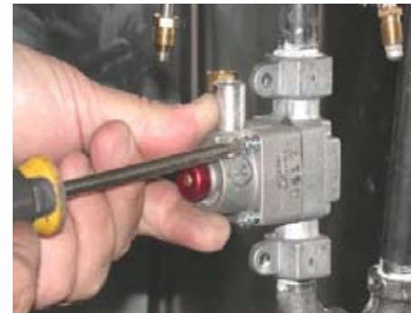
4. Remove the screws from the safety head.
