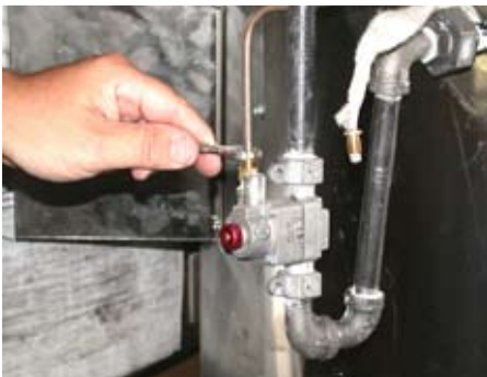
3. Using a 7/16" wrench, remove the brass fitting from the pilot gas line.
