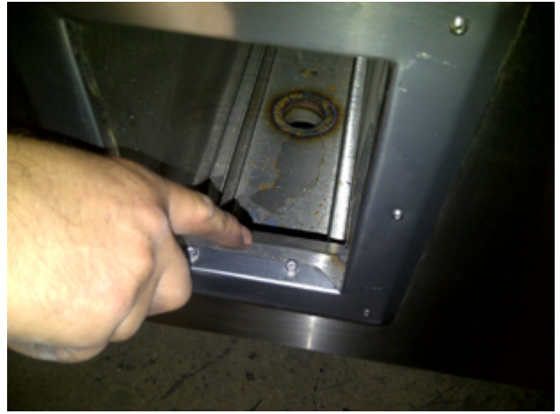
2 REMOVE SCREWS HOLDING SINK.
