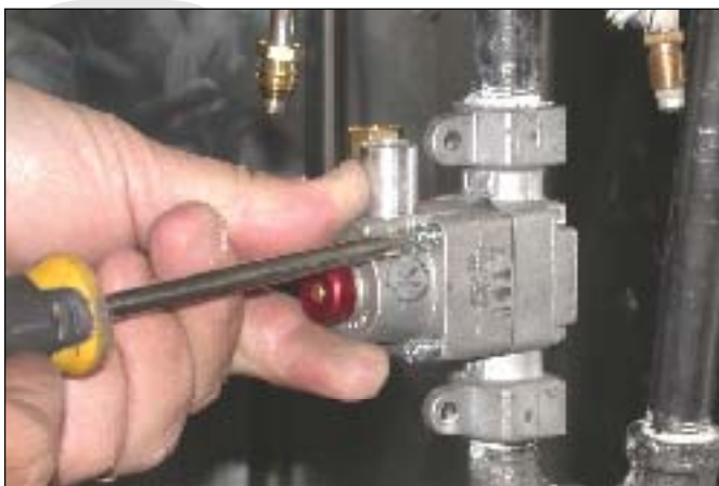
9 Mount the safety head and replace the screws
