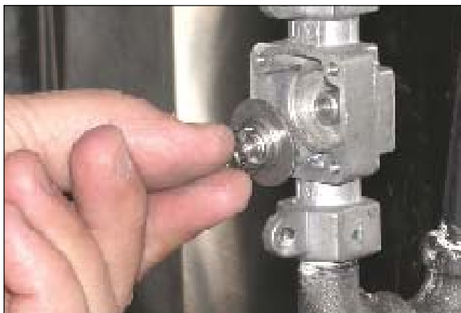
6 Remove and replace the spring/magnet assembly
