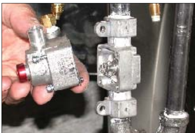
4 Remove the safety head
