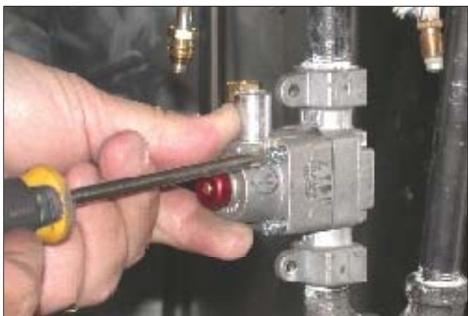
3 Remove the screws from the safety head
