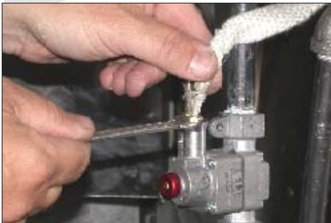
11 Thread the thermocouple fitting into the body by hand. When you can no longer tighten by hand, use a 3/8" wrench to make snug. A 1/4" turn after finger tightening is recommended. Do not overtighten as it will damage the control. Turn on gas, check for leaks, and relight pilot.
