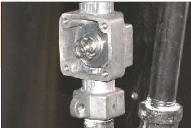
7 New spring/magnet assembly installed
