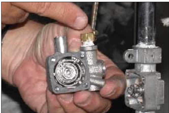
5 Remove brass adaptor safety head and install on the new head
