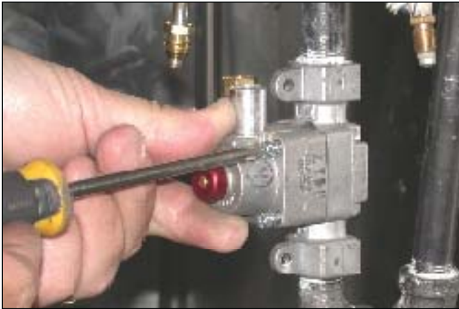
3 Remove the screws from the safety head
