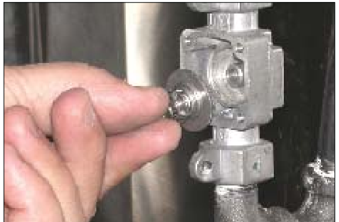
6 Remove and replace the spring/magnet assembly
