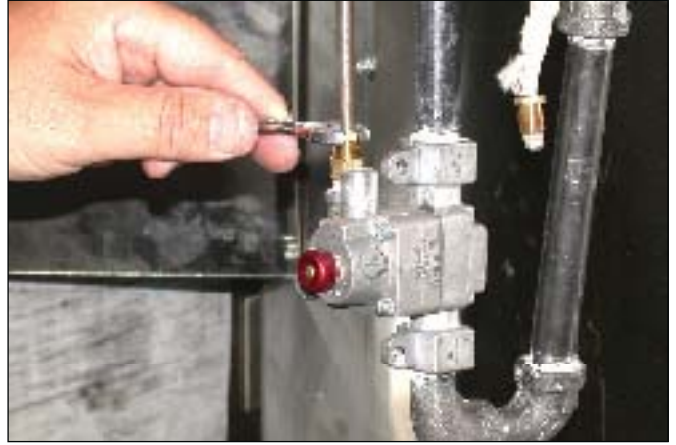
2 Using a 7/16" wrench, remove the brass fitting from the pilot gas line
