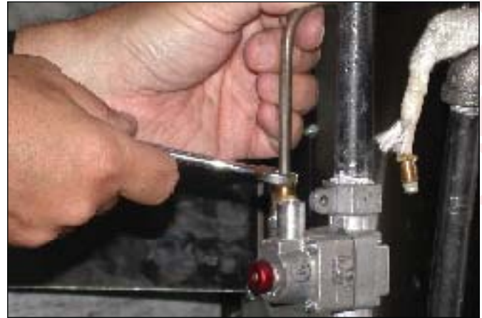
10 Carefully thread the brass fitting from the pilot gas line into the body and tighten using a 1/4" wrench.
