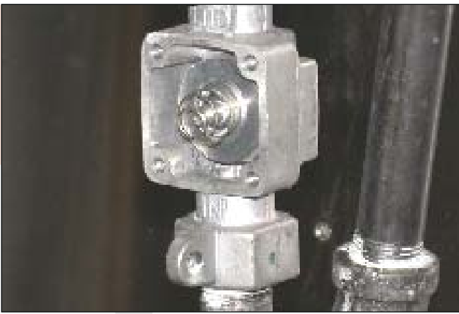
7 New spring/magnet assembly installed
