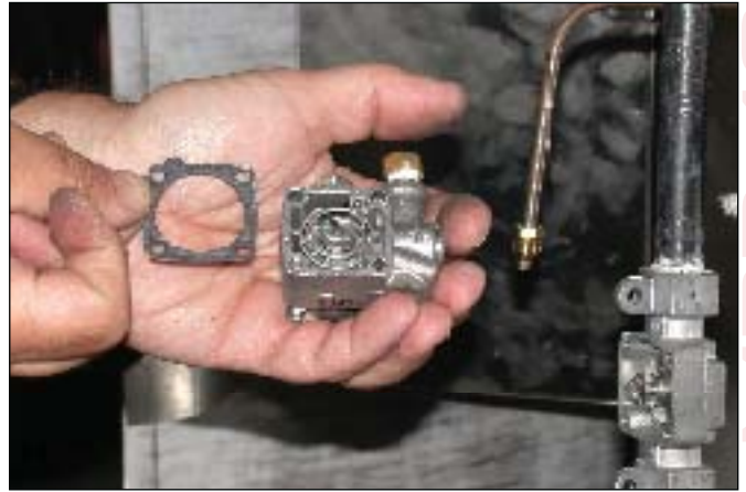
8 Install the new safety head with the new gasket provided. Clean old gasket material first.
