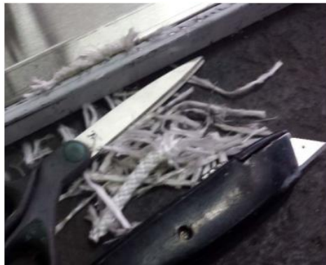
Figure 2 – After Cutting existing door gasket
